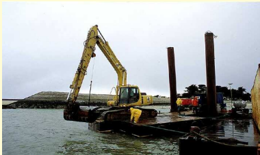
Backhoe in harbour.
